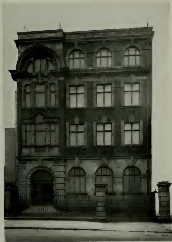
FRONTAGE OF THIRD LABORATORY OF SCHOOL.
